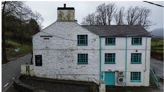
The north-eastern facing side elevation where there is a clear and distinct difference between the main original 19 th century building and the 20 th century addition to the rear.
