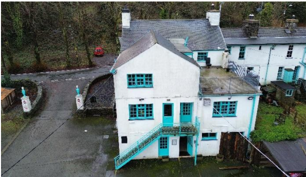
Rear elevation with the gable wall of the dining lounge and the flat roofed terrace on the right with the rear of the Brondanw terrace in view. Brondanw Estate pilasters set back at junction splay to highway on the left.
