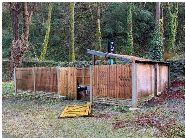
Bin, recycling and storage compound adjacent to car park.
